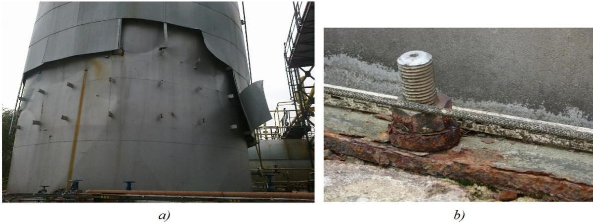
**Fig. 2: A) View of Places with the Largest Deformations; B) Display of Rips of the Tank Anchorage**
